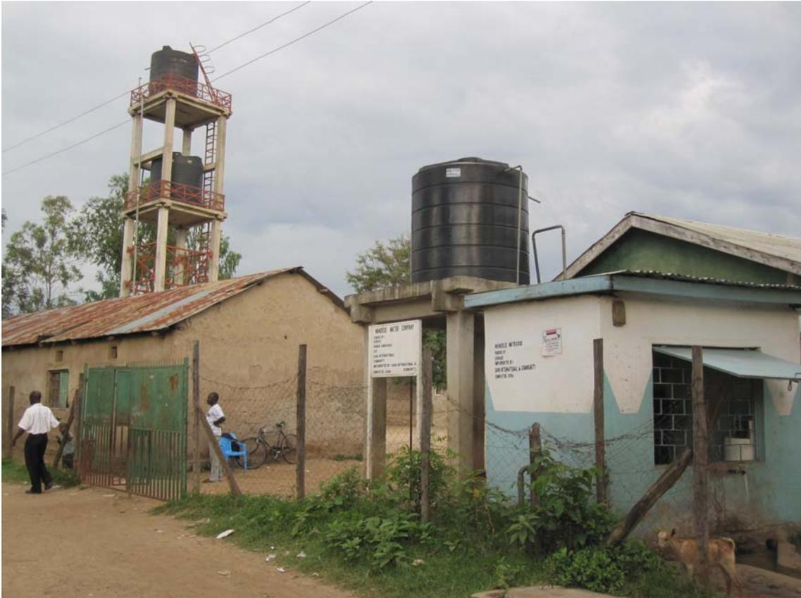
*Photo 1* The Wandiege pumping station-cum-water kiosk (right) and the two 10,000 litres storage tanks [photo: Dick Foeken, 2012]
