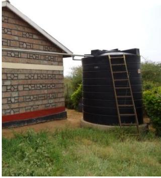
**Photo1: RWH using plastic tanks**
