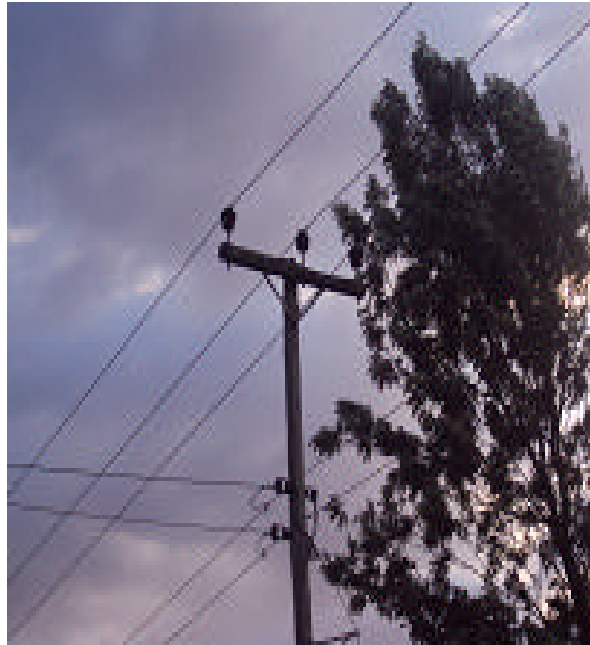
Fig. 3: High and Low voltage power lines interfered by an inappropriately planted urban tree
