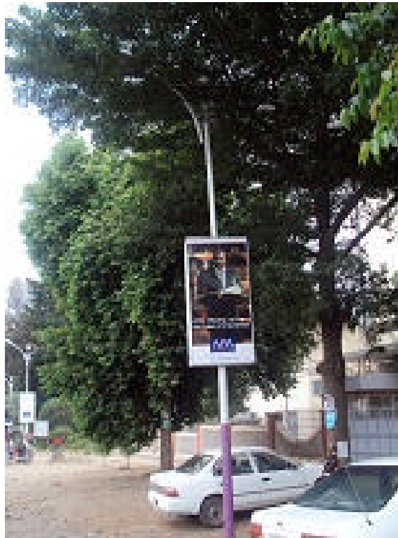
Fig. 1: A Street light covered by tree branches
