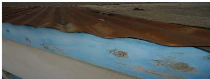
Figure 4. Corroded galvanized roofing sheet near a highway in Nairobi, Kenya
